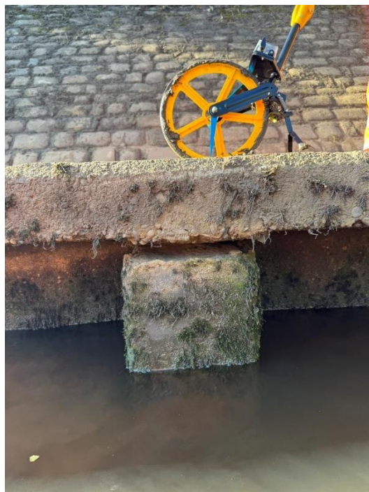
04 Gap between the capping beam and pile. The capping beam not bearing onto the pile. Steel reinforcement exposed on the top of the pile.
