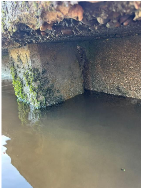
20 Aggregate visible at the surface of the capping beam. Spalling at the back of the pile with exposed and corroded steel reinforcement.
