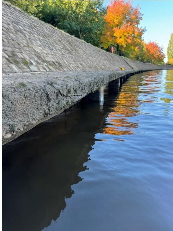
75 Capping beam in ok condition.
