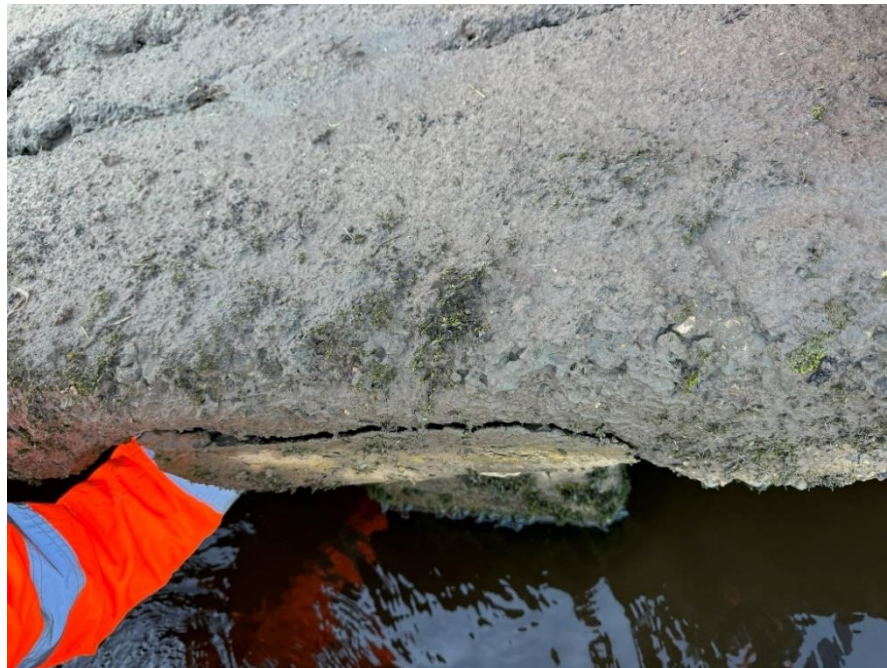
76 Cracking and loose concrete on the side of the capping beam above the pile.
