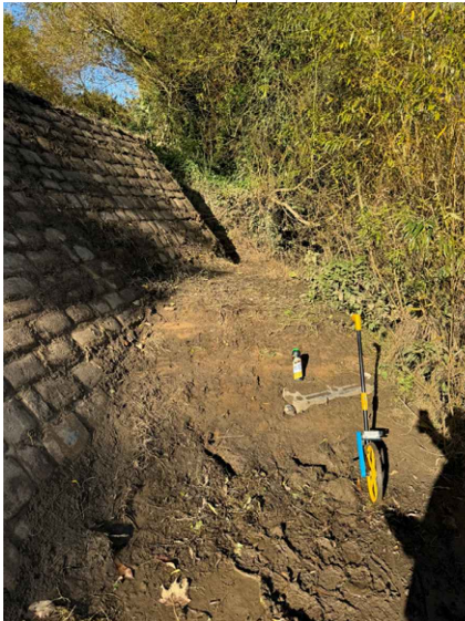
Chainage 0-5m Overgrown vegetation and large build up of earth at the base of the pitched stone embankment.
