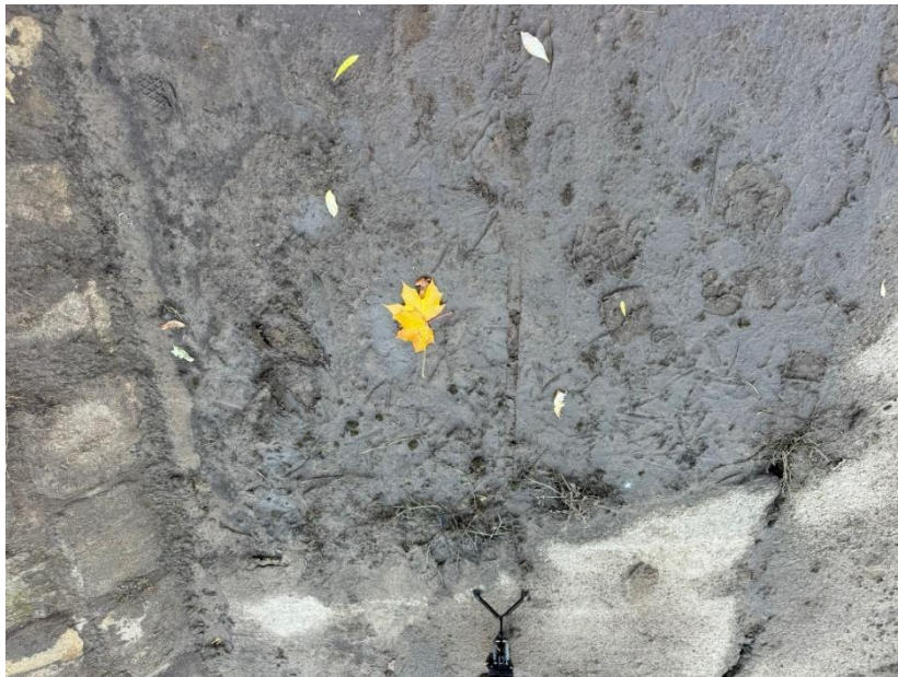
62 Build-up of silt on top of the concrete path. Large crack in the slab propagating from the capping beam to the bottom of the pitched stone.
