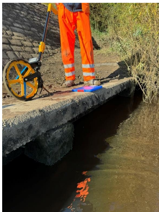
02 Capping beam at the furthest point along the riverbank, approximately 270m upstream from the Scarborough Rail Bridge.
