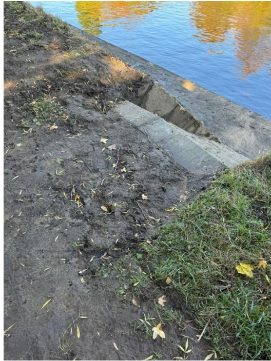
115 Top of embankment steps. The top steps are out of place.
