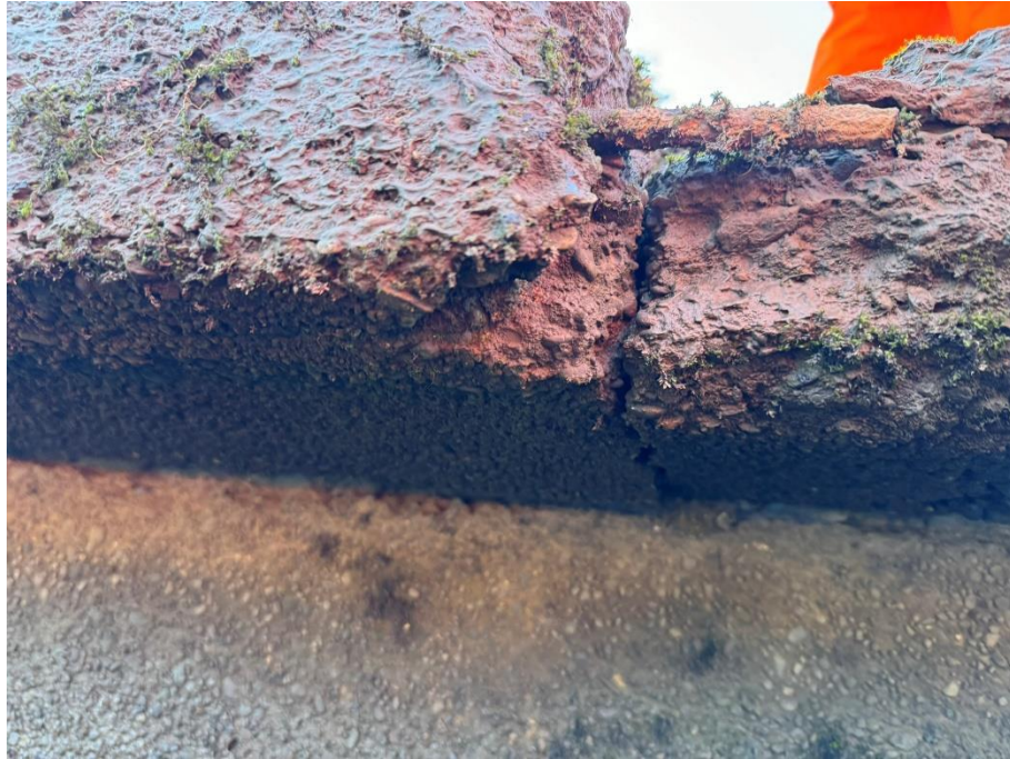
81 Large section loss in capping beam with exposed steel reinforcement. Crack through the width of the capping beam.
