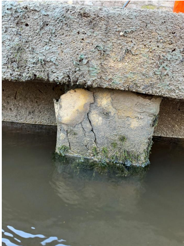
45 Cracking on the top of the pile, concrete is loose.
