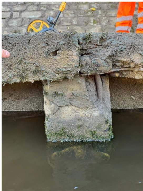
44 Concrete spalling on the side of the concrete capping beam and top of the pile. Spalling has exposed the steel reinforcement. The reinforcement is corroded.
