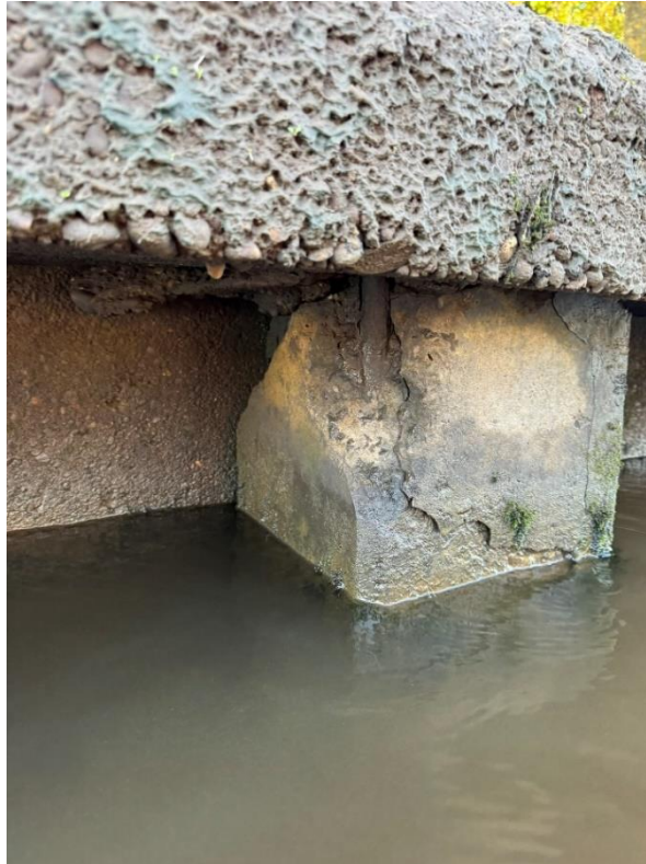
37 Cracking at the top of the pile. Spalling on on the top of the concrete pile, exposed steel reinforcement.
