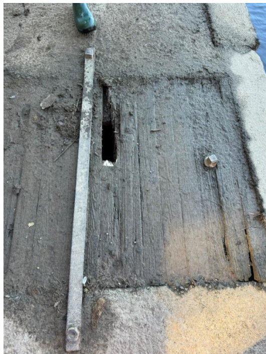
88 Timber service cover in poor condition, timber is rotting.
