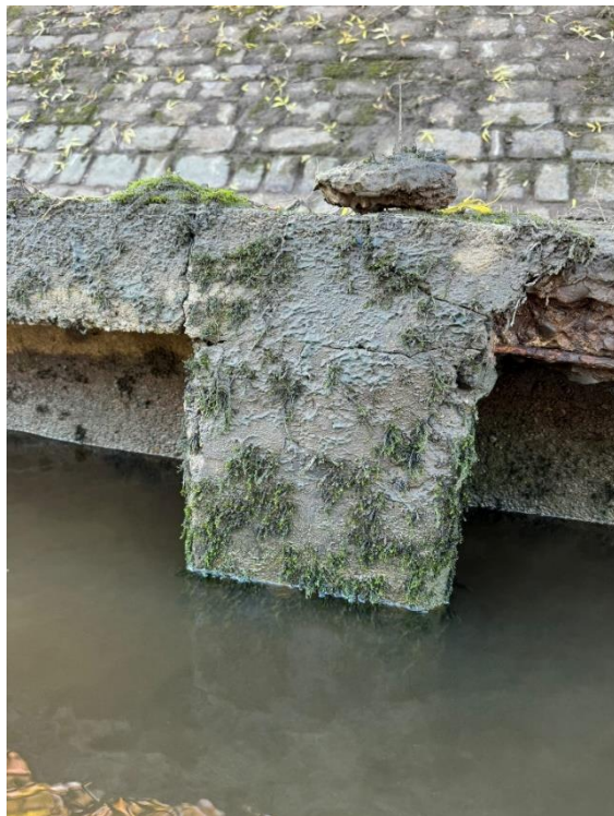
34 Concrete spalling and exposed corroded steel reinforcement in the capping beam. Surface cracks on the pile.
