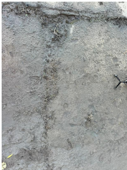
86 Crack in the concrete path, propogating from the capping beam to the pitched stone.
