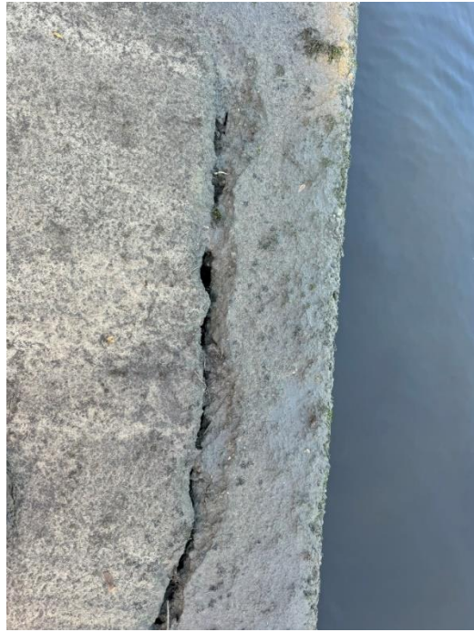
75 Large crack between the capping beam and concrete path.
