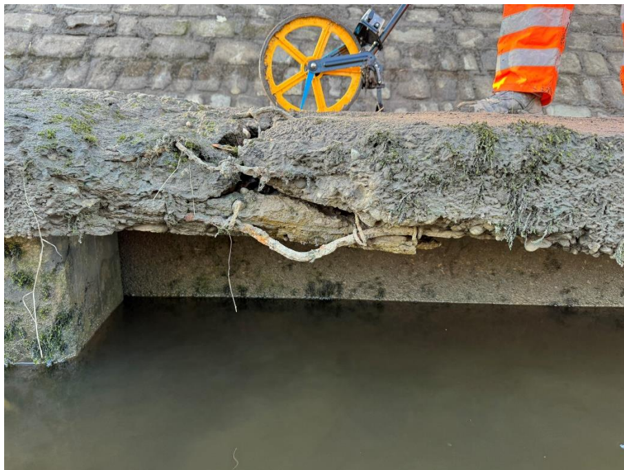
28 Severe cracking in the capping beam, with concret spalling. Exposed, deformed and corroded steel reinforcement.
