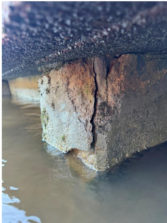
62 Spalled concrete at the top of the pile, with corroded steel reinforcement exposed.
