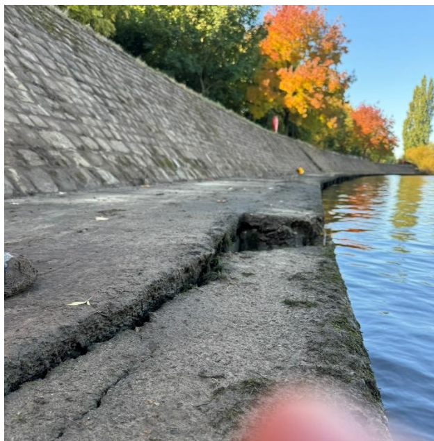
78 Top of the capping beam at point of failure.
