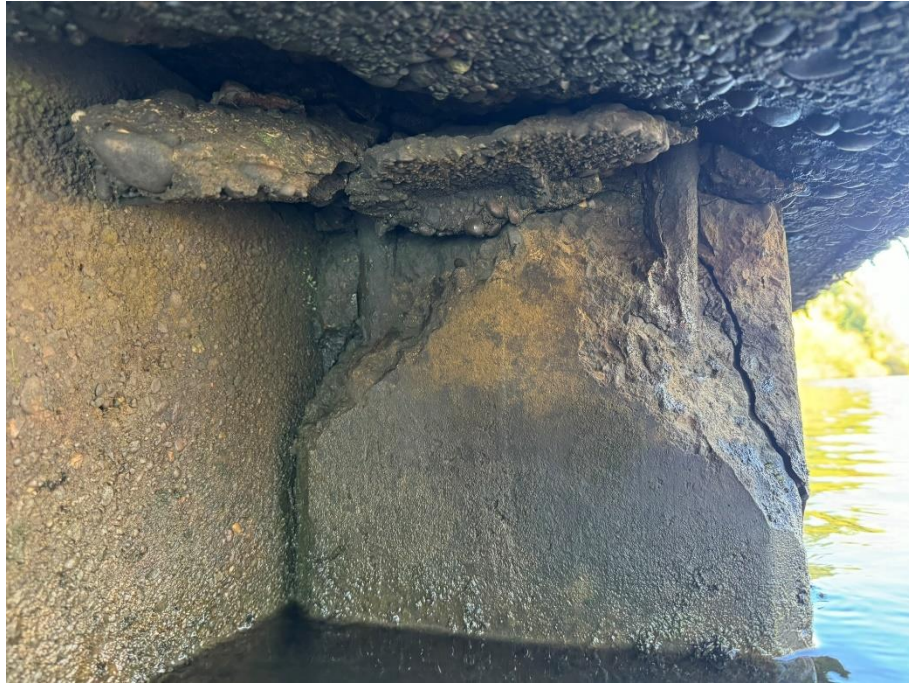
39 Cracking at the top of the pile. Spalling on on the top of the concrete pile, exposed steel reinforcement.
