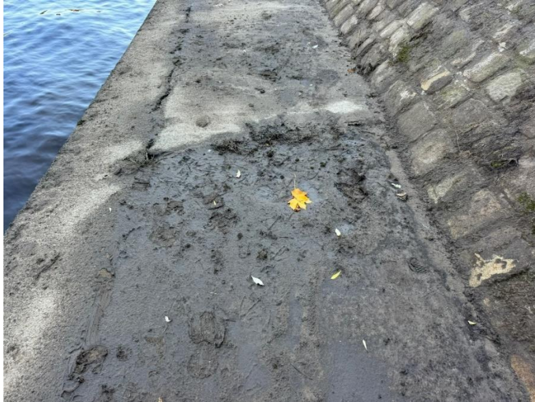
61 Build-up of silt on top of the concrete path. Large crack in the slab propagating from the capping beam to the bottom of the pitched stone.
