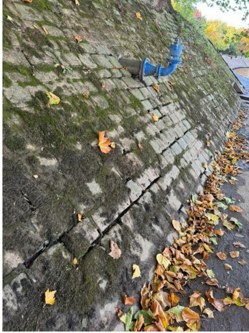
101 Missing mortar between stones on the pitched stone embankment.
