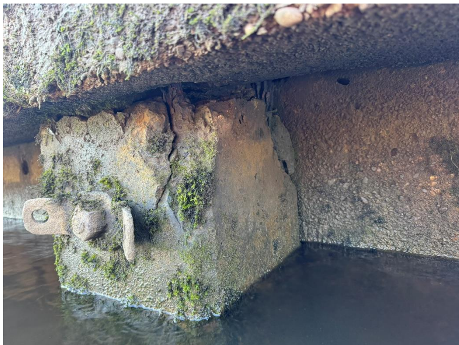
50 Spalling of concrete at the top of the pile. Corroded steel reinforcement bars are exposed.
