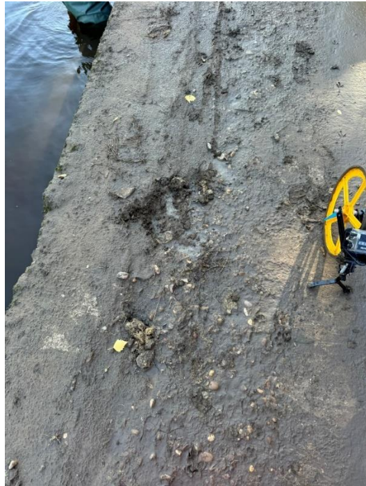
09 Loose aggregate on concret slab surface.
