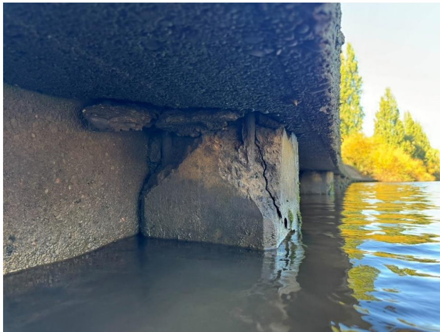
38 Cracking at the top of the pile. Spalling on on the top of the concrete pile, exposed steel reinforcement.
