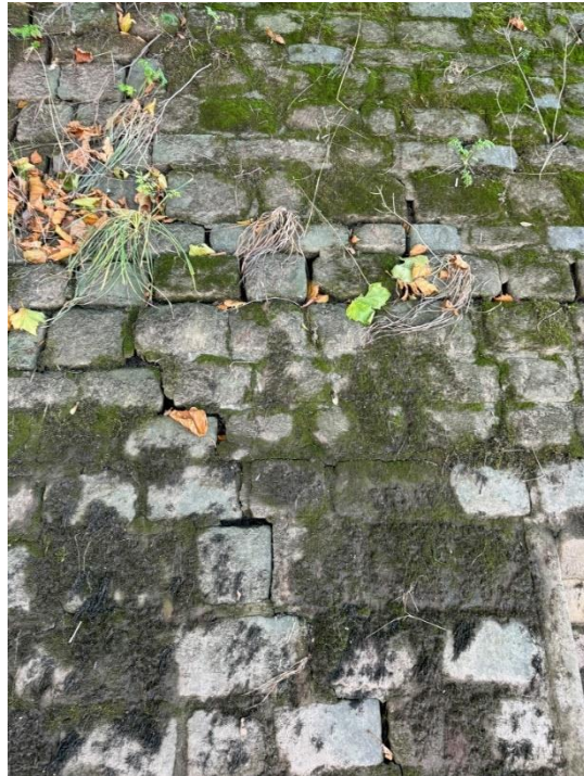
105 Missing mortar between stones on the pitched stone embankment.
