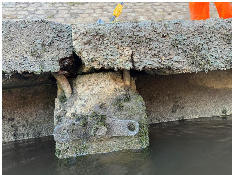
52 Spalling of concrete at the top of the pile and underside of the capping beam. Corroded steel reinforcement bars are deformed and exposed.
