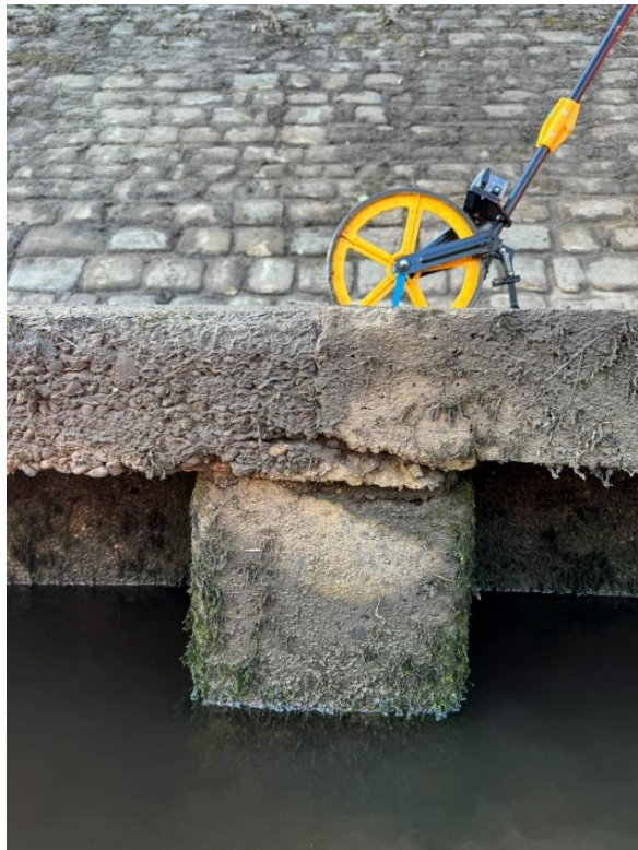
12 Cracking on the bottom of the capping beam.
