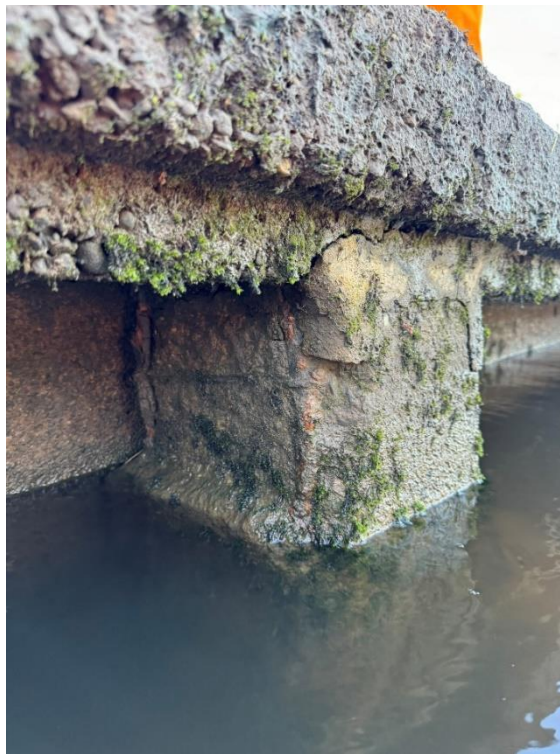
84 Concrete spalled and exposed steel reinforcement at the top of the pile.
