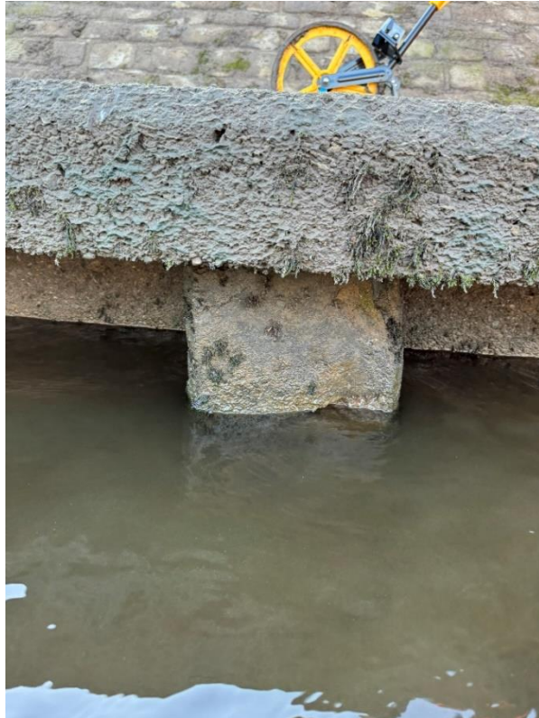
61 Capping beam and pile in ok condition.
