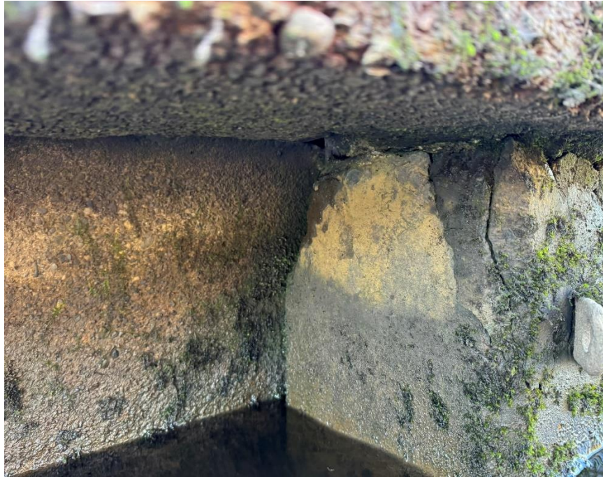
51 Spalling of concrete at the top of the pile. Corroded steel reinforcement bars are exposed.
