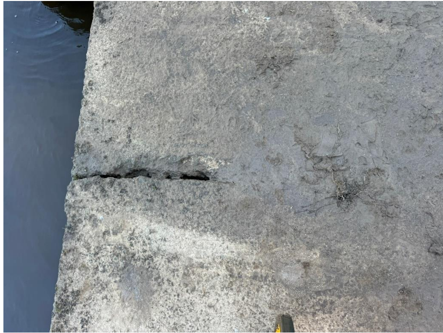
79 Crack in the concrete capping beam.
