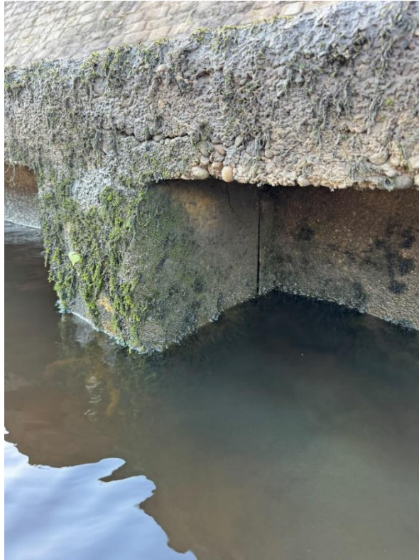
17 Aggregate visible at the surface of the capping beam. Crack at the back of the pile.
