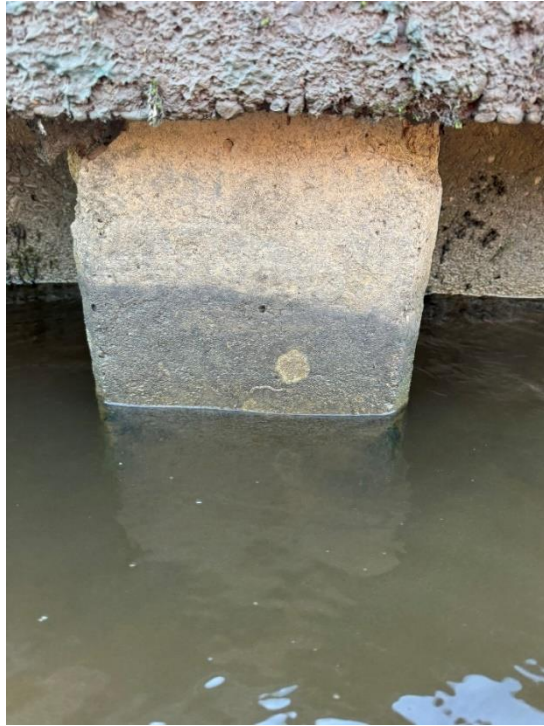
63 Minor spalling to top corners of the pile.
