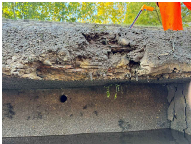
Chainage 26m Concrete spalling and exposed steel reinforcement on the capping beam. Additionally concrete spalling is visible on the reinforced concrete pile.
