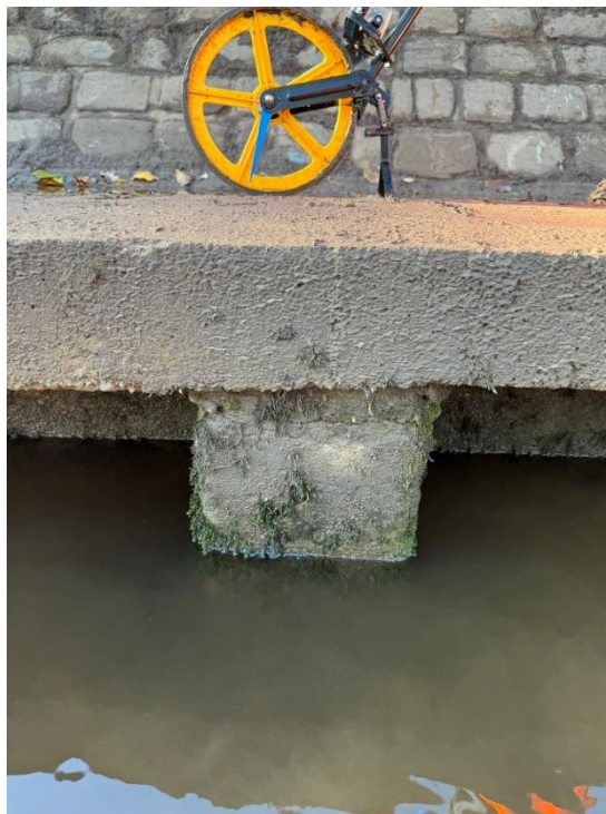
10 Photo of capping beam in ok condition. Cracks in the top of the pile.
