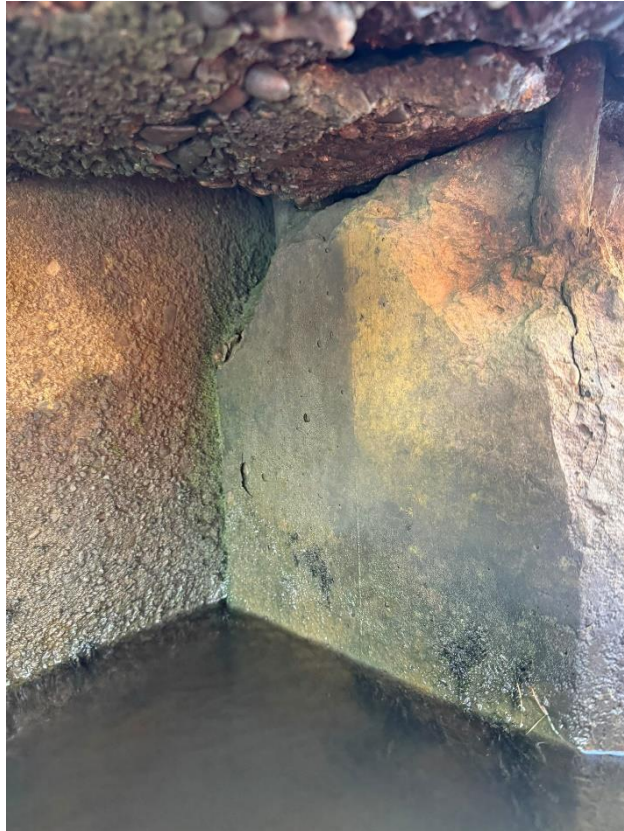
43 Spalling on on the top of the concrete pile, exposed steel reinforcement.
