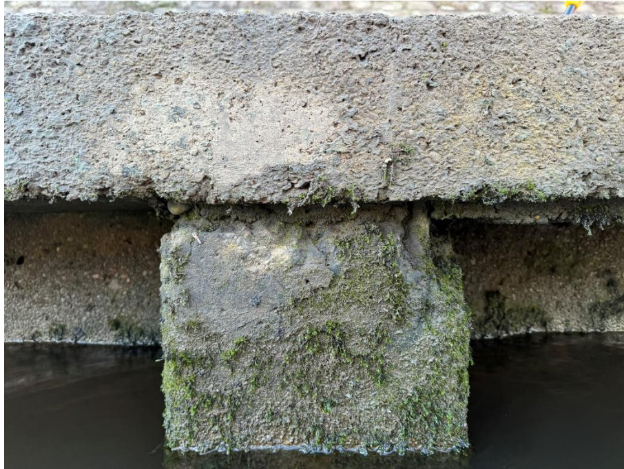
53 Spalling to top corner of the concrete pile, with exposed steel reinforcement.
