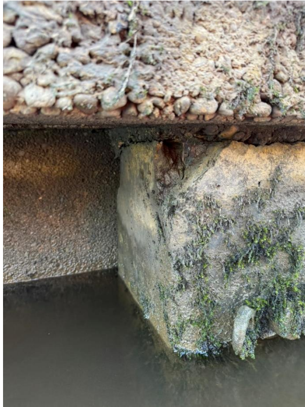
35 Spalling on on the top of the concrete pile, exposed steel reinforcement.
