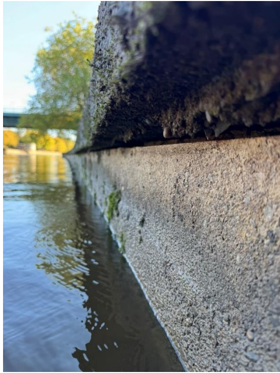
87 Concrete retainnig wall in good condition.
