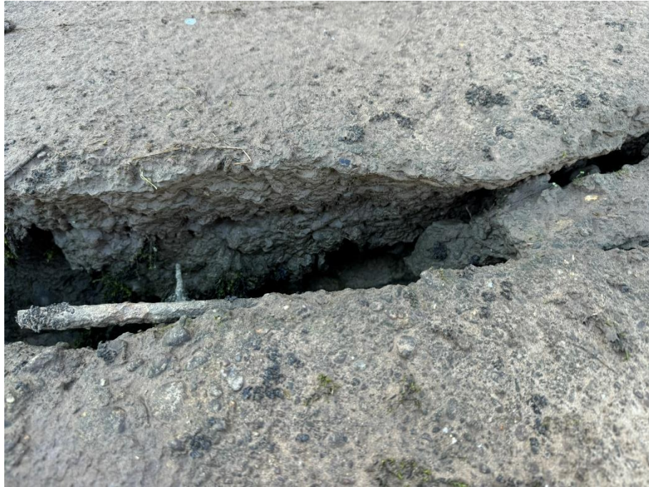
77 Large gap between the capping beam and concrete path. Exposed steel reinforcement.
