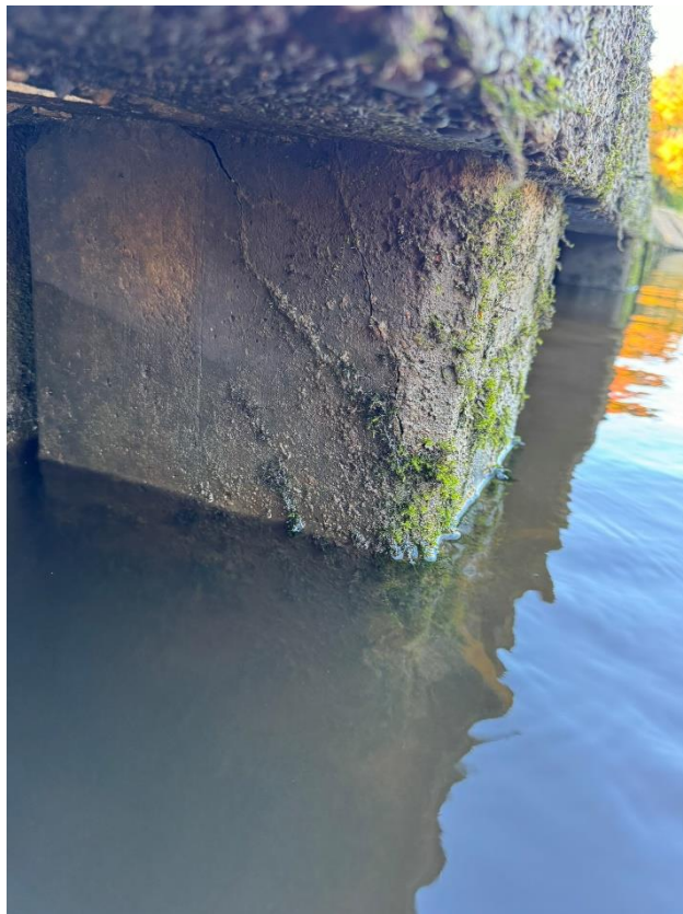
82 Surface cracking at the top of the pile.
