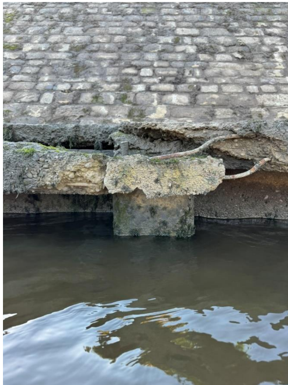
64 Failed capping beam, no longer sufficiently supported and breaking away from concrete path. Large cracking and deformed steel reinforcement exposed in the capping beam and pile.
