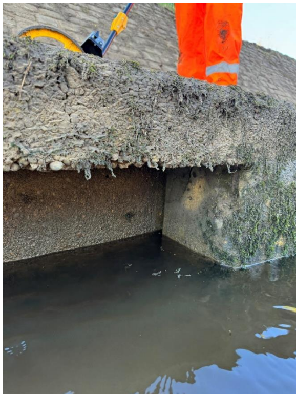
18 Aggregate visible at the surface of the capping beam. Gap between the retaining wall and pile.
