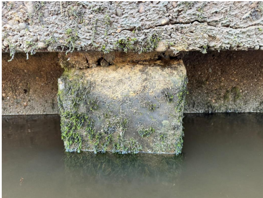
26 Close up of concrete spalling at the top of the pile with exposed corroded steel reinforcement.
