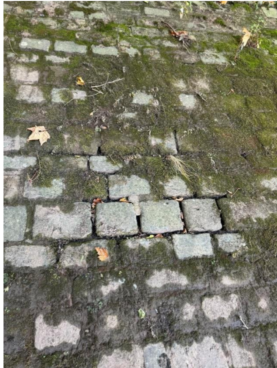
99 Missing mortar between stones on the pitched stone embankment.
