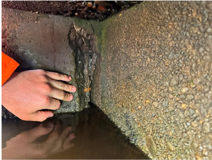
21 Spalling at the back of the pile with exposed and corroded steel reinforcement.
