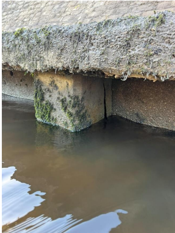
19 Aggregate visible at the surface of the capping beam. Crack at the back of the pile.
