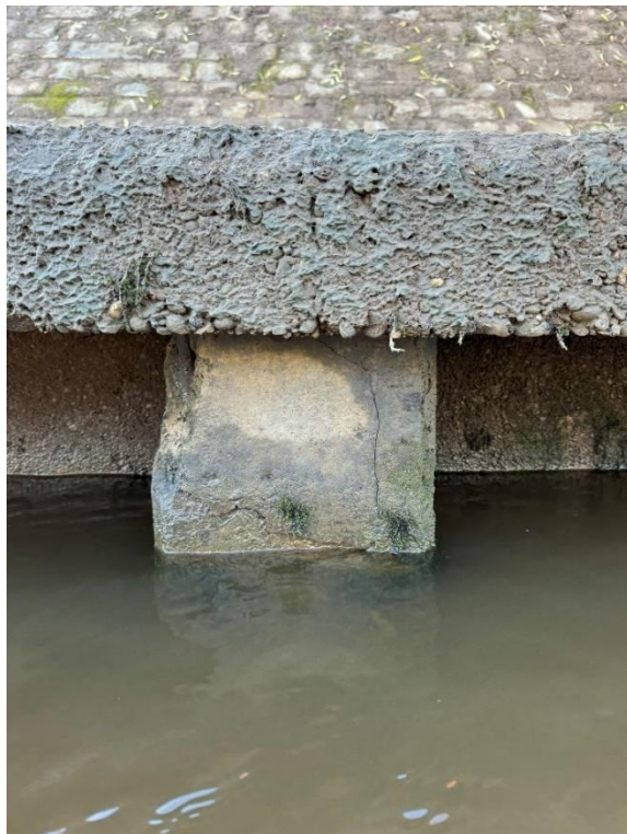
36 Cracking at the top of the pile. Spalling on on the top of the concrete pile, exposed steel reinforcement.
