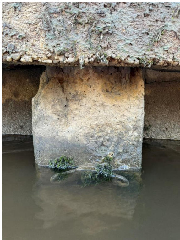
42 Spalling on on the top of the concrete pile, exposed steel reinforcement.
