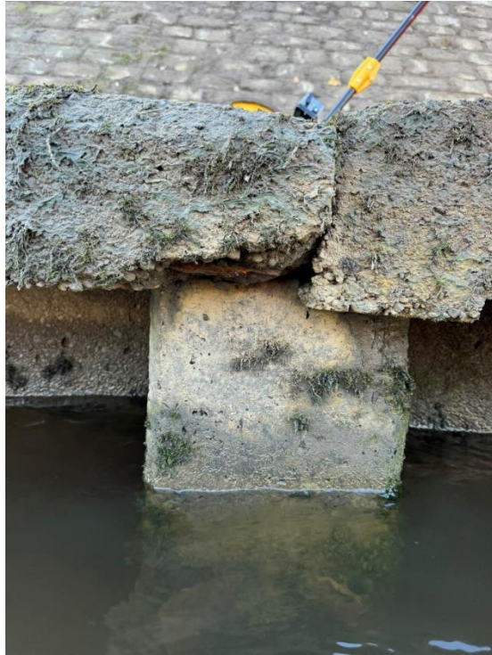
47 Spalling of concrete to the underside of the capping beam. Corroded steel reinforcement is exposed.
