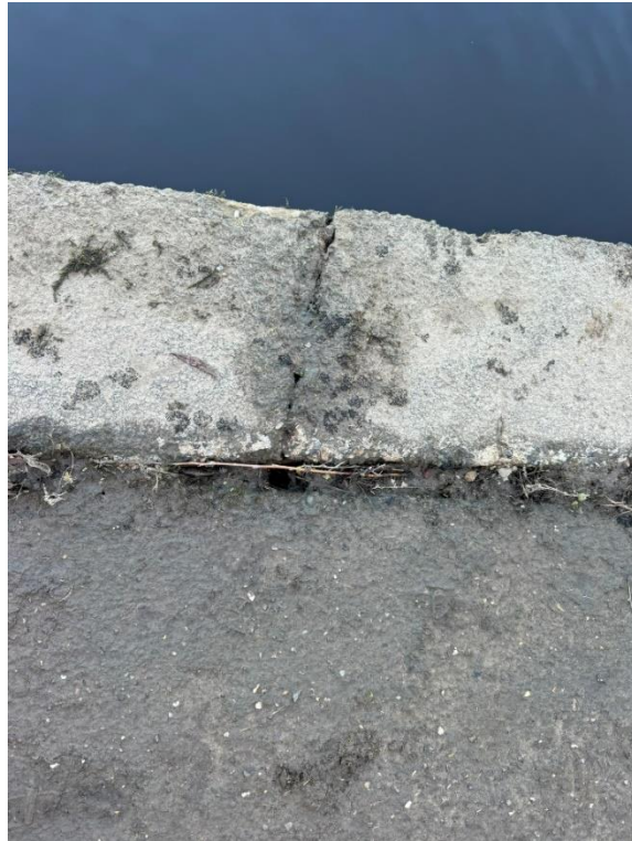
85 Crack in the top of the capping beam.
