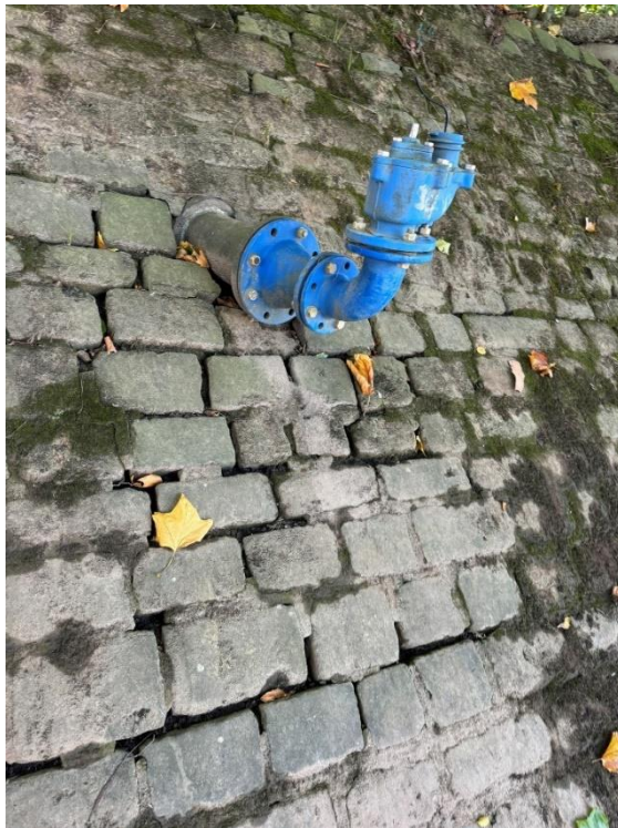
102 Missing mortar between stones on the pitched stone embankment around a service valve.
