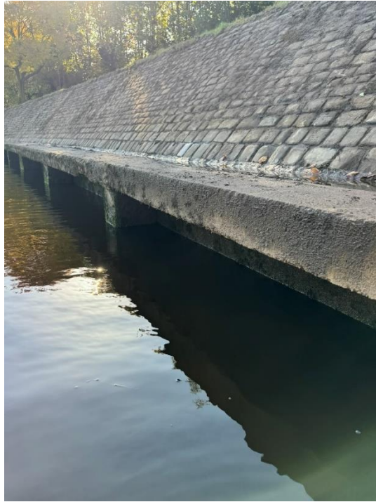
11 Photo of capping beam in ok condition.
