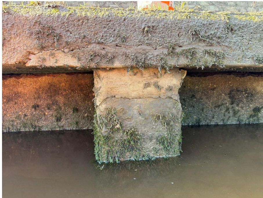
05 Cracking at the top of the pile and side of the capping beam. Retaining wall is ok.
