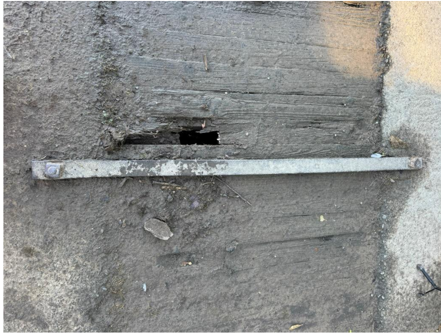
87 Timber service cover in poor condition, timber is rotting.
