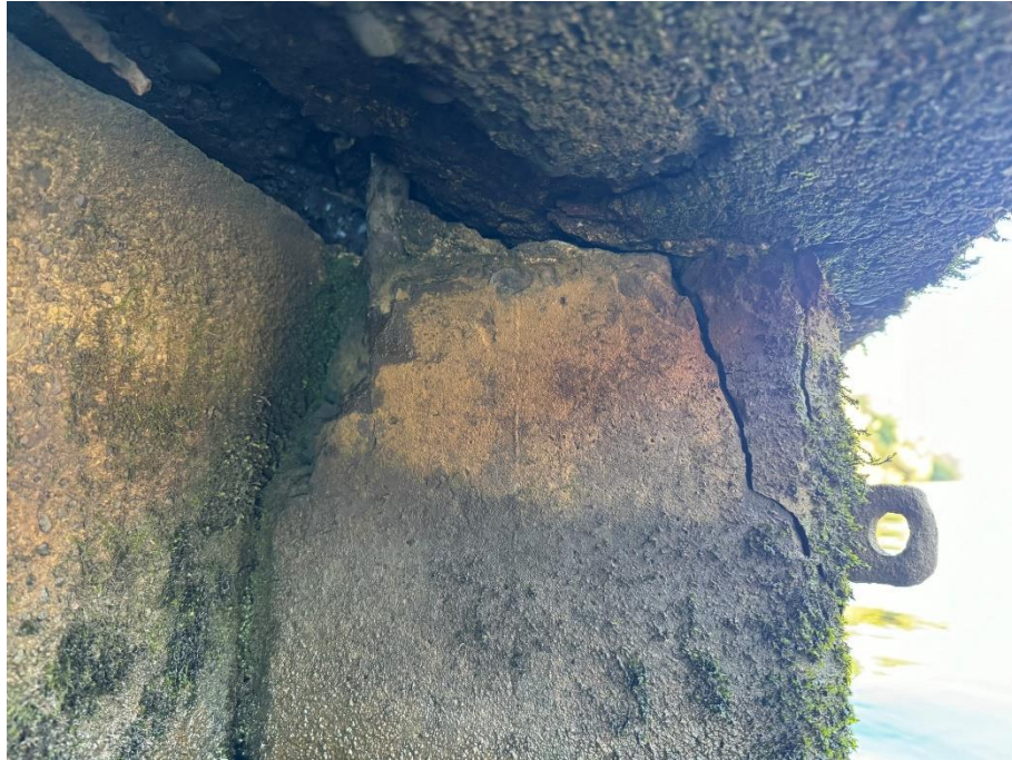
49 Spalling of concrete at the top of the pile. Steel reinforcement bars are exposed.
