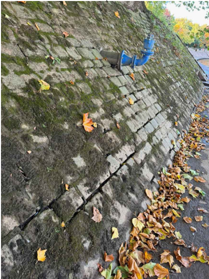
Chainage 255m Missing mortar and loose stones in the pitched stone embankment.
