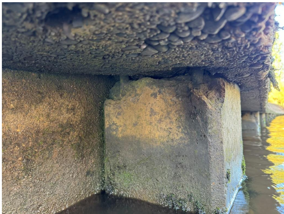
40 Spalling on on the top of the concrete pile, exposed steel reinforcement.
