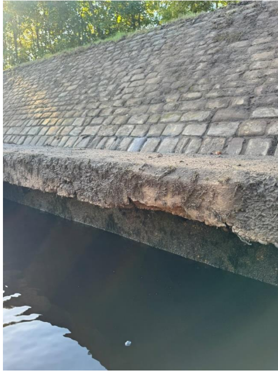
13 Photo of concrete spalling on the bottom of the capping beam.
