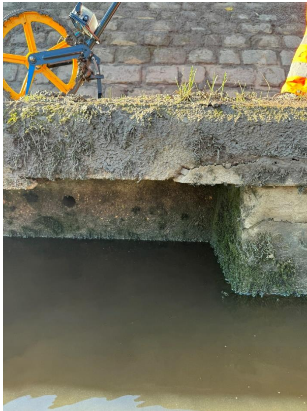
08 Cracking in capping beam and top of the pile.
