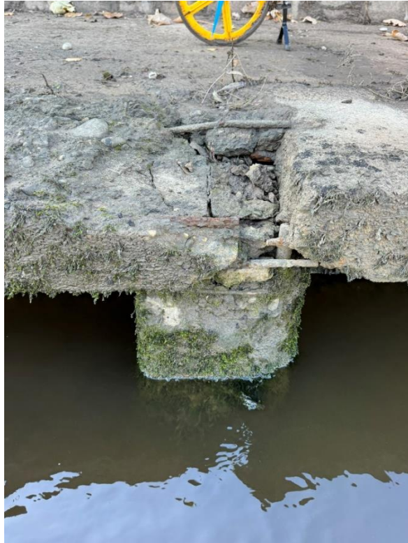
55 Spalled and loose concrete on top of the capping beam and pile, with corroded and deformed steel exposed.
