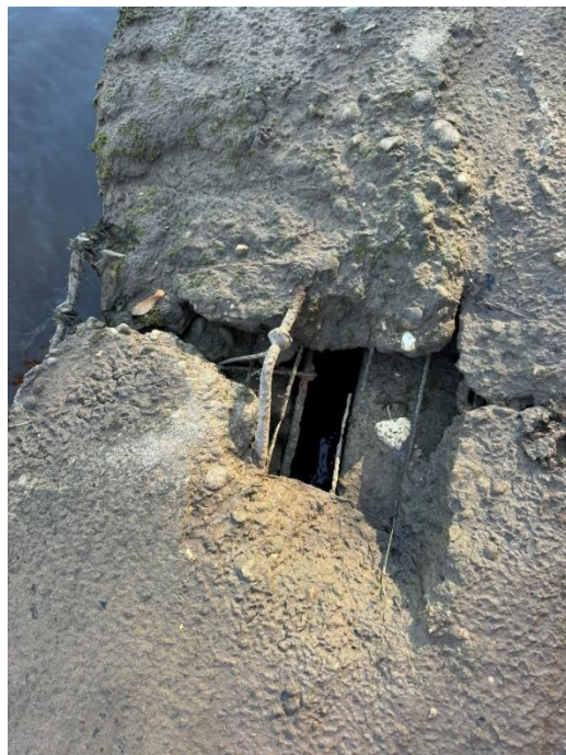
10 Loss of section on the capping beam, concrete spalled and broken away exposing deformed steel reinforcement. Can see through the capping beam to the top of the pile underneath.
