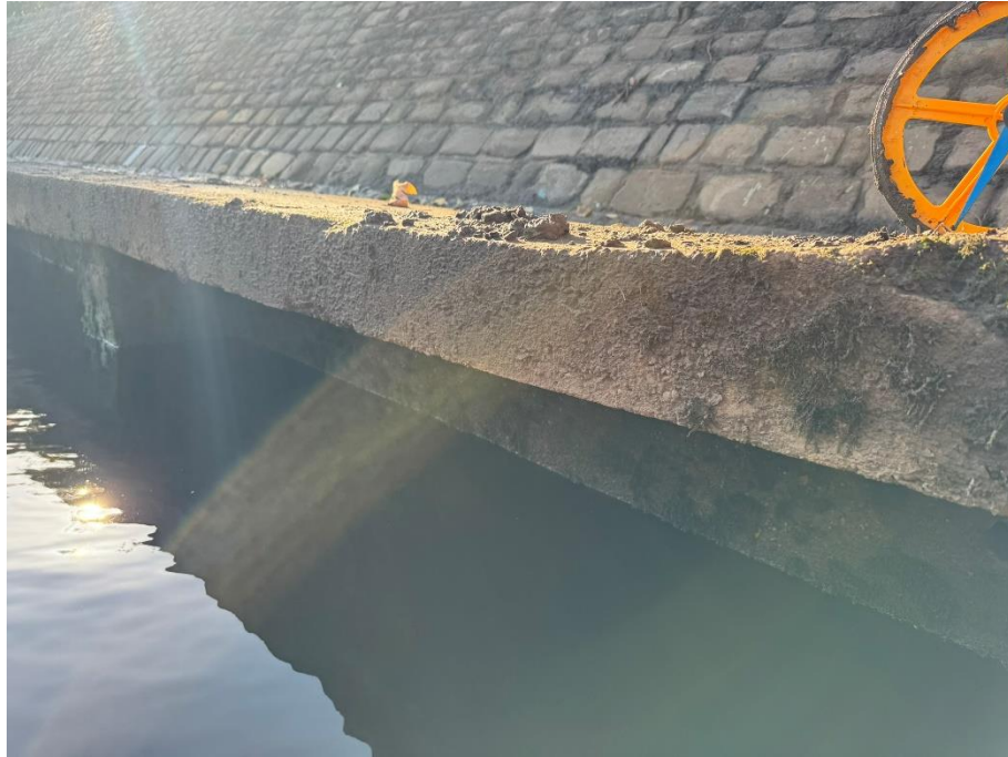
07 Photo of capping beam in ok condition.
