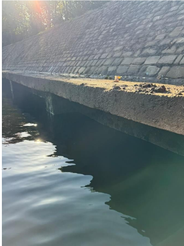
09 Photo of capping beam in ok condition.
