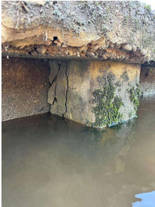
22 Spalling at the back of the pile and underside of the capping beam.
