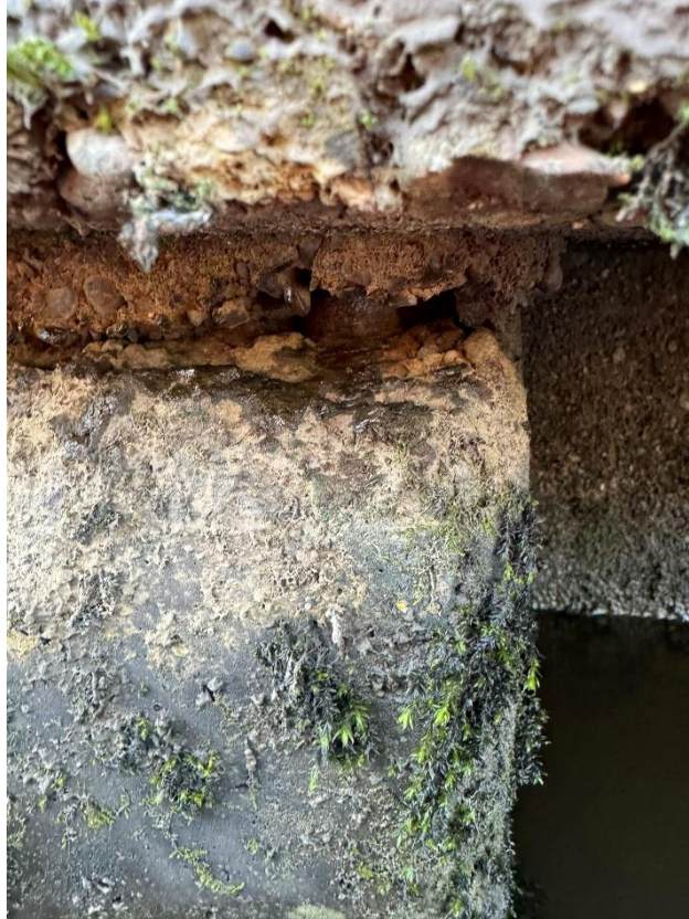
25 Close up of concrete spalling at the top of the pile with exposed corroded steel reinforcement.
