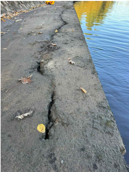
Chainage 76m Large crack between the concrete path and reinforced concrete capping beam. The capping beam is tilting about its minor axis towards the river.
