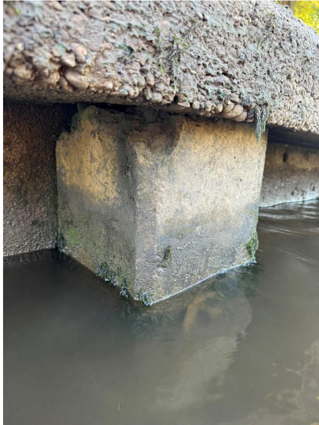
41 Spalling on on the top of the concrete pile, exposed steel reinforcement.
