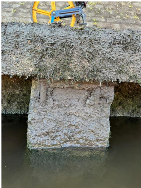
56 Spalled concrete at the top of the pile, with corroded steel reinforcement exposed.
