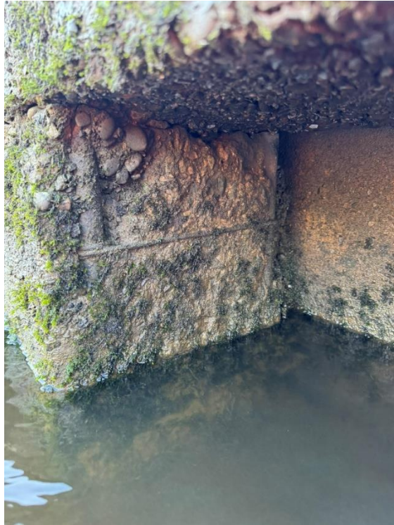
83 Concrete spalled and exposed steel reinforcement at the top of the pile.
