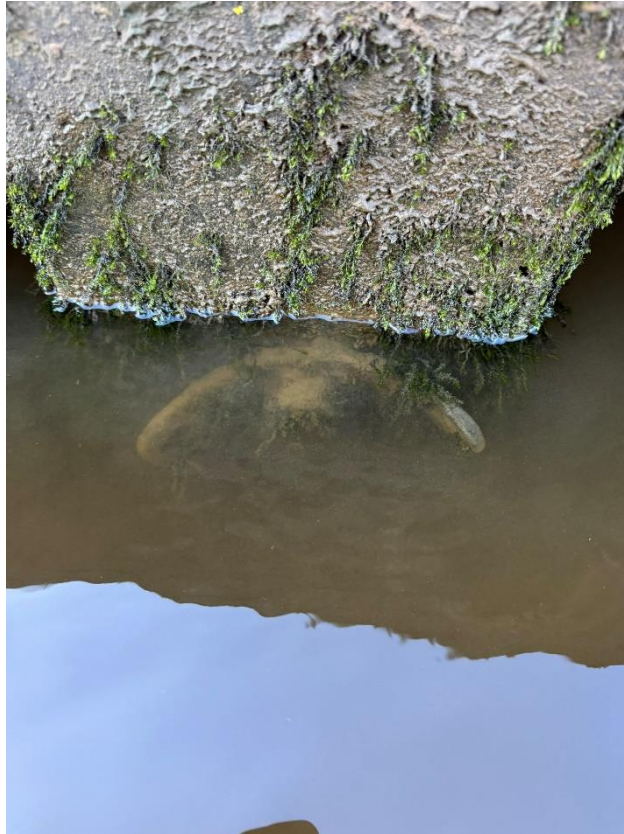
27 Steel anchor threaded through concrete pile.
