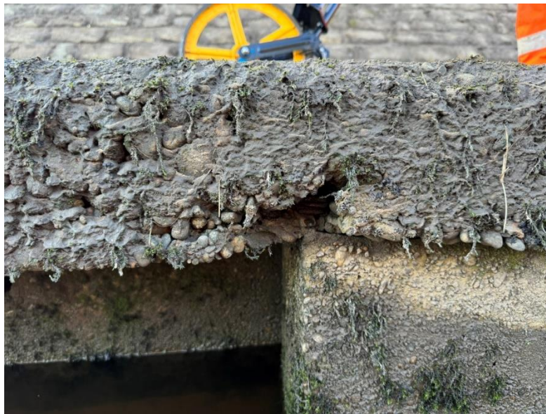
14 Spalled concrete under the capping beam with exposed and corroded steel reinforcement.
