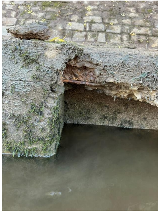
33 Concrete spalling and exposed corroded steel reinforcement in the capping beam. Surface cracks on the pile.
