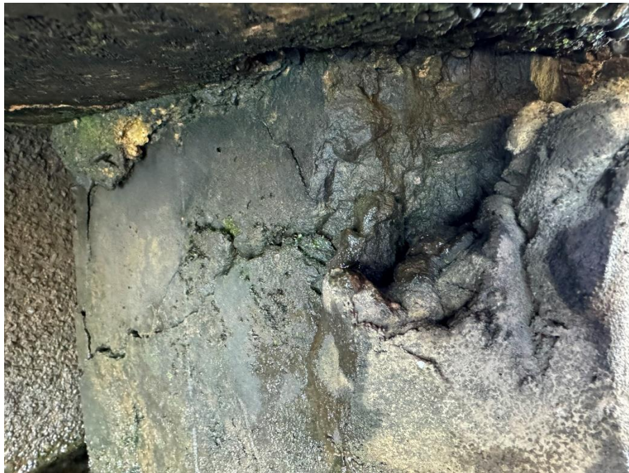
46 Spalling of concrete at the top of the pile.
