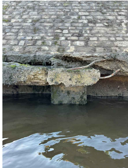
Chainage 176m Failed capping beam, no longer sufficiently supported and breaking away from concrete path. Large cracking and exposed steel reinforcement in the capping beam.
