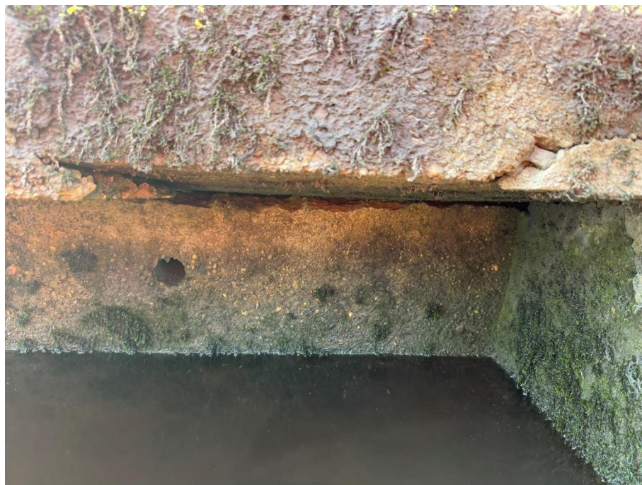
06 Cracking in the capping beam. Retaining wall okay.
