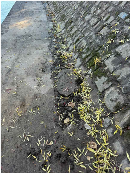
Chainage 55m Void and broken up concrete slab at the base of the pitched stone retaining wall. Areas of slab loose at the surface.
